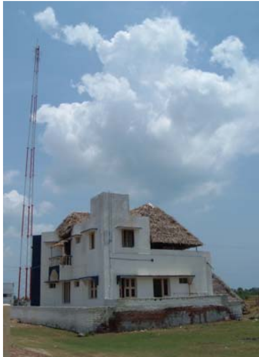
Enabling wireless communications: The communication tower at the NCRC head office
