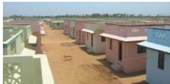
The Tarangambadi site, ready for possession
