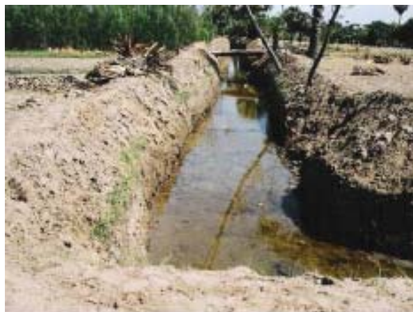
Clean, de-silted canal
