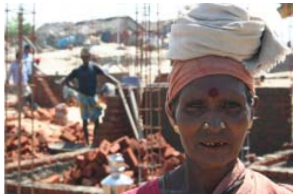
Networking construction labourers
