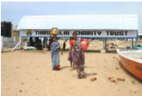
Water treatment plant
